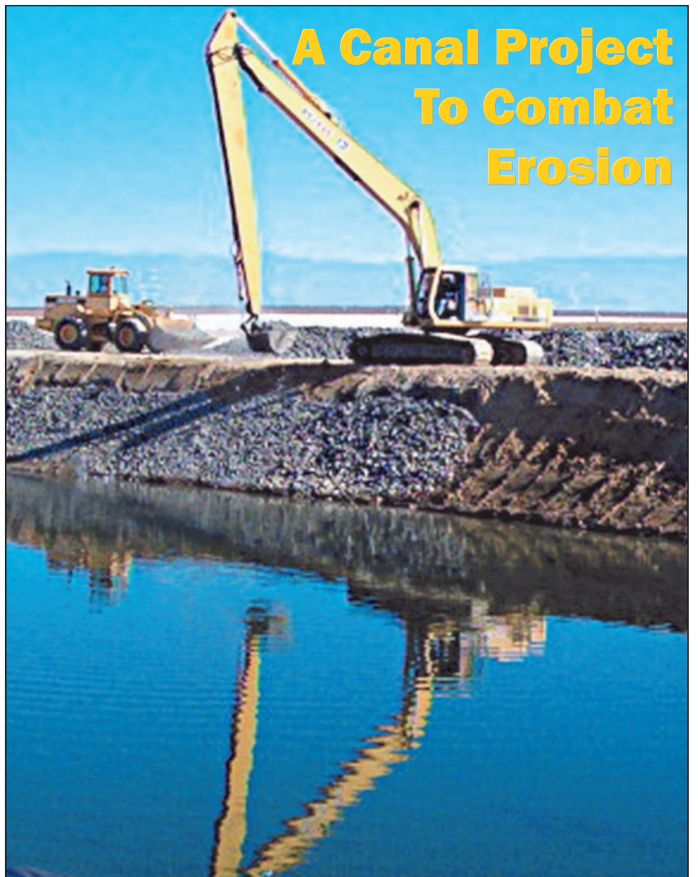
Friant Water Authority An unlined Friant-Kern Canal section along Lake Woollomes, the canal's re-regulating reservoir southeast of Delano, has received 8,000 tons of rip-rap material on its inside banks to protect the canal from erosion due to currents and wave action. Similar work is being done on the reservoir's inside embankments.
