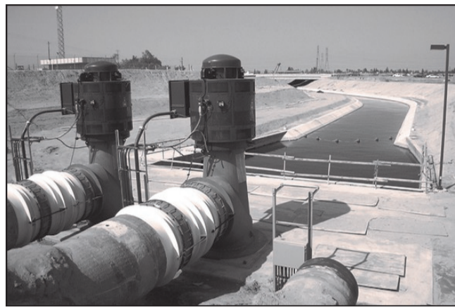
The Cross Valley Canal in Kern County
