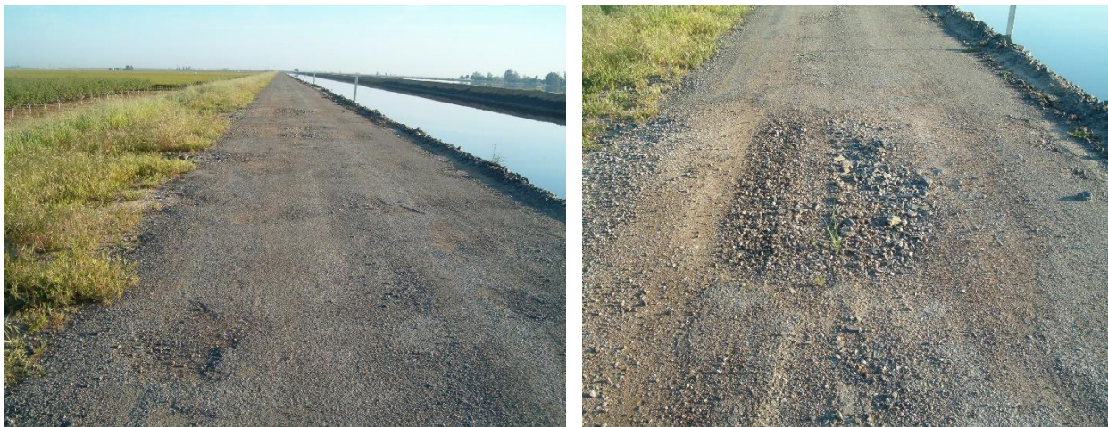
Photo of Existing Conditions
