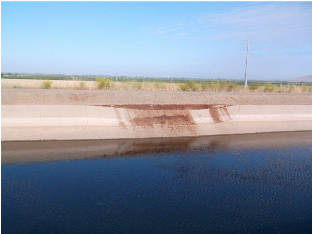
Photo of Existing Conditions
