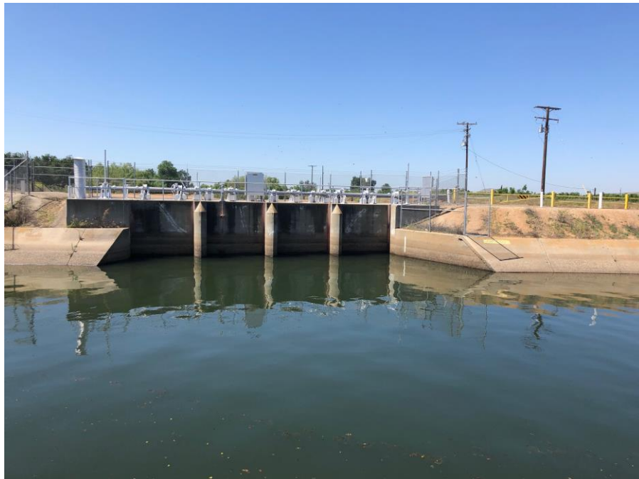
Photo of Existing Conditions MP. 69.42 Waste way Structure
