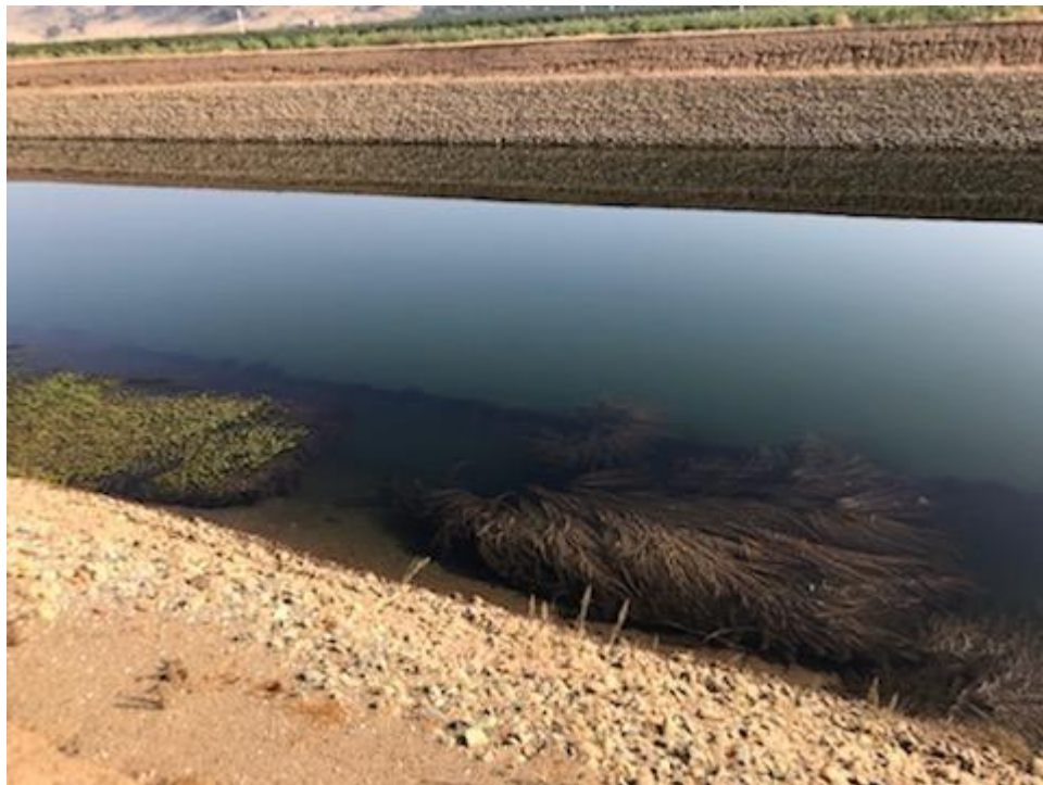
Photo of Existing Conditions MP 48.60
